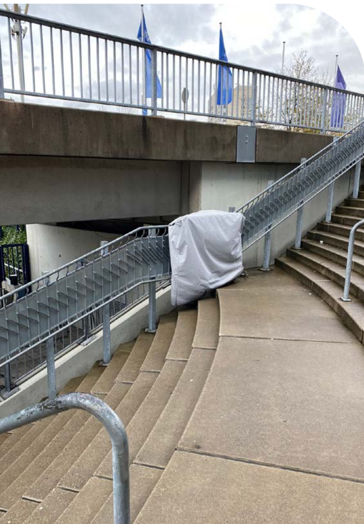
Image 12 | An external, non-enclosed stairlift at Arena AufSchalke
