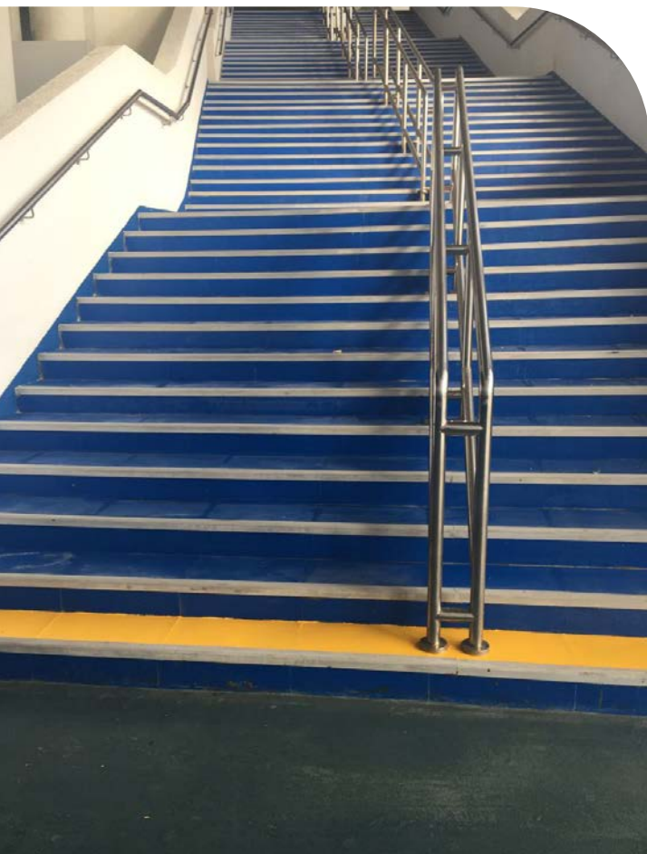
Image 14 | A stairway with uniform steps, handrails and contrasting step edges at Fisht Olympic Stadium, Sochi
