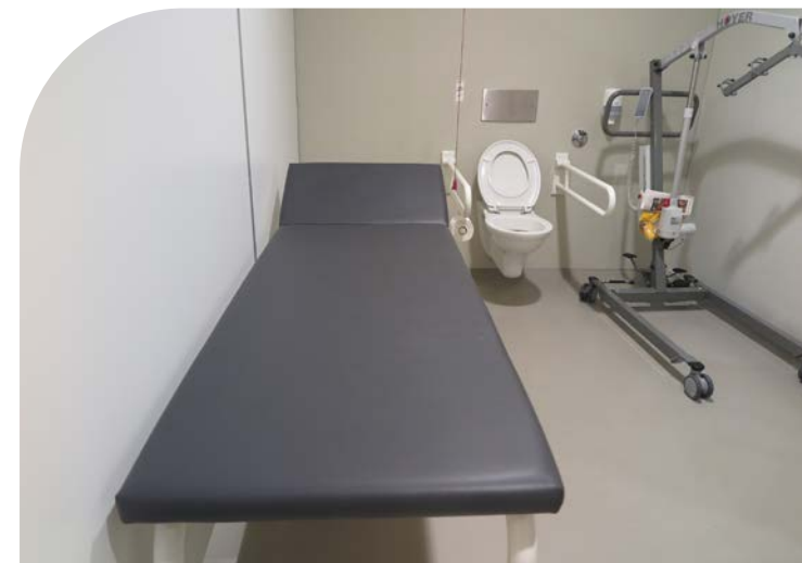
Image 22 | An example of a Changing Places toilet facility with a peninsular toilet at Munich Football Arena
